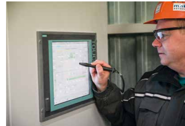
Dirk Schubert, master electrical engineering technician and specialist responsible for the flue gas treatment system in the field of operations
